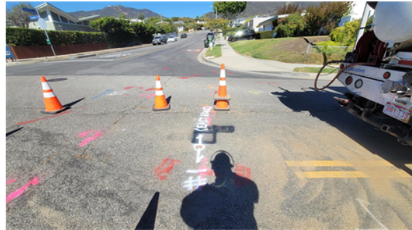
SITE PHOTO - FACING NORTH
