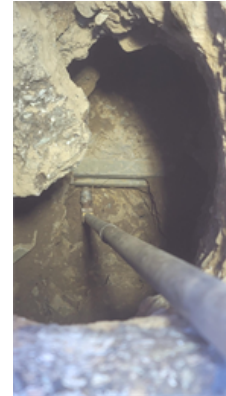
TEST HOLE - UTILITY - FACING NORTH
